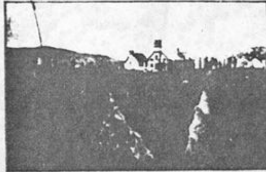
The dump at Schreiber on the C. P. R. just a few minutes after the water began to wash through under the track. The dump is 85 feet in height. Schreiber churches show in the background. The culvert under this dump was not large enough to carry the water, the creek coming through there being so swollen by the heavy rain.
